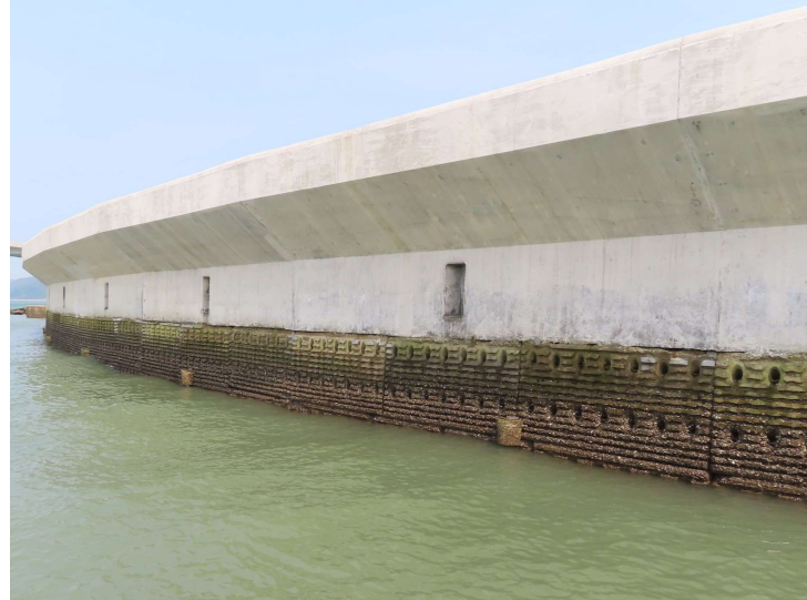
General View of Vertical Eco-shoreline
