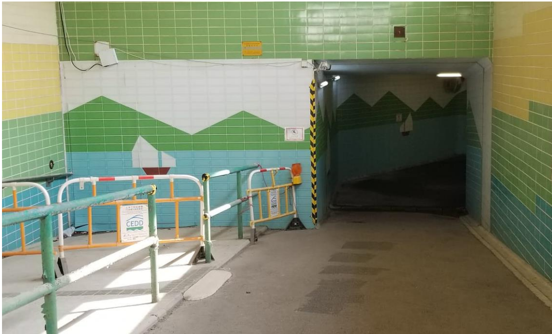
Photo 3 - Erection of site hoardings in unobtrusive colours
